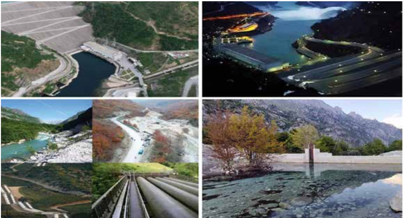
Fierza Hydroelectric Power Station and Small Hydropower Plants
